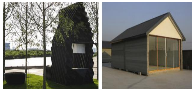
Fig. 4: (a) First 3D printed house (taken from Dus Architects [50]) (b) 3D printed house (taken from P. Wu et al [3])
