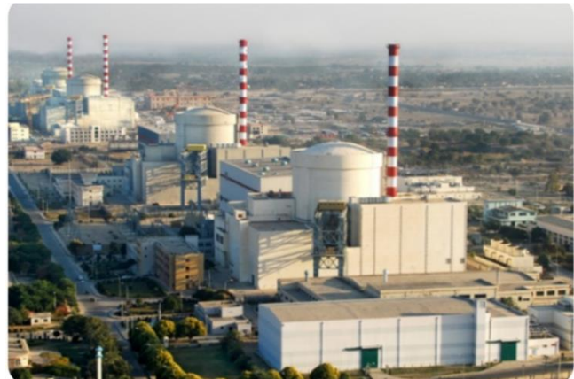
Fig. 1: Aerial view of Nuclear Power Plants in Mianwali
