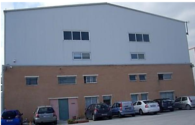
Fig. 1: Concrete-steel frame (Hybrid building) https://taxonomy.openquake.org/index.php/terms/hybrid-lateral-load-resisting-system-lh
