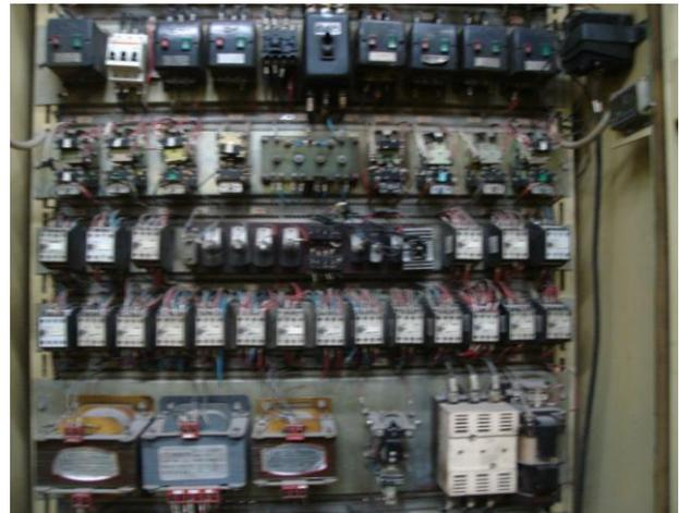
Figure 3. Snapshot of relays to control the operation of machine.
