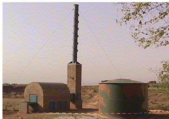
Incinerator at ARL.
